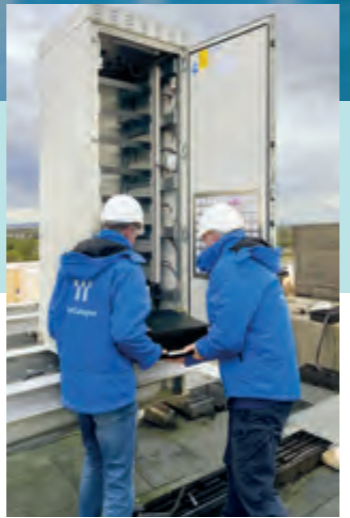
Installation of the system technology and lithium batteries
