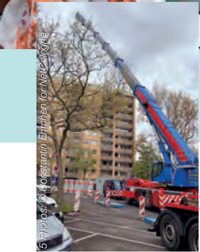
Smooth installation on site; the outdoor cabinets are set down and installed on an existing platform using a crane
